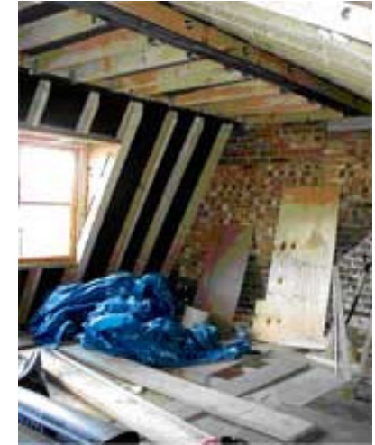
Interior of New Dormer Roof Extension
