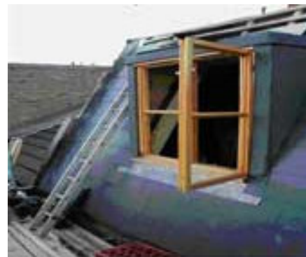
New Dormer Roof
