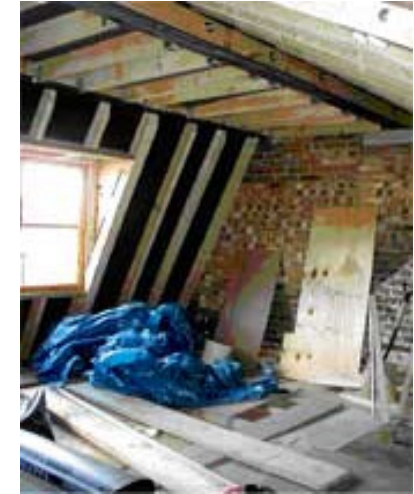
Interior of New Dormer Roof Extension
