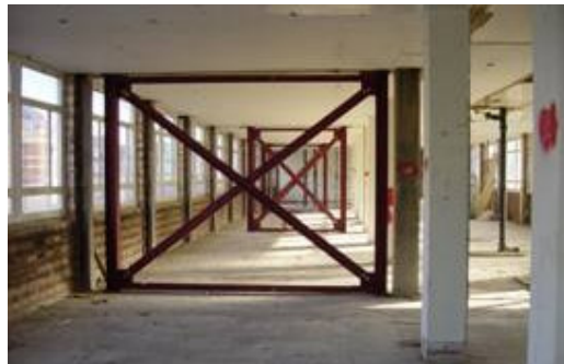
New Structural Steelwork Cross Bracing
