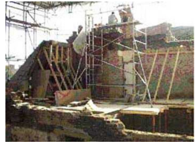
Demolition and Reconstruction of the Levels 4 & 5 Floors and Roofs
