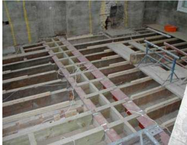
Typical Strengthening of Existing Floors
