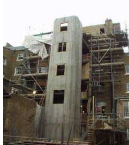
Construction of New Lift Shaft, Stair Core & Rear Extension
