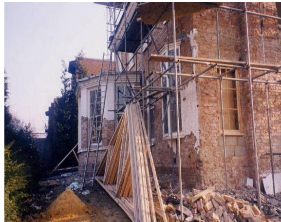
Front of House (Work in Progress)
