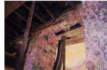
Propping to New Opening
