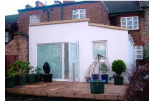
Completed Rear Extension
