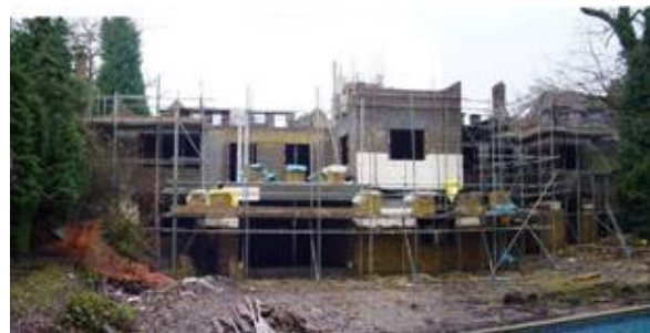
Construction of Rear Elevation
