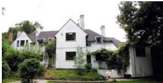
Original Rear Elevation
