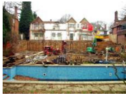
Rear Elevation (Excavation for New Basement)
